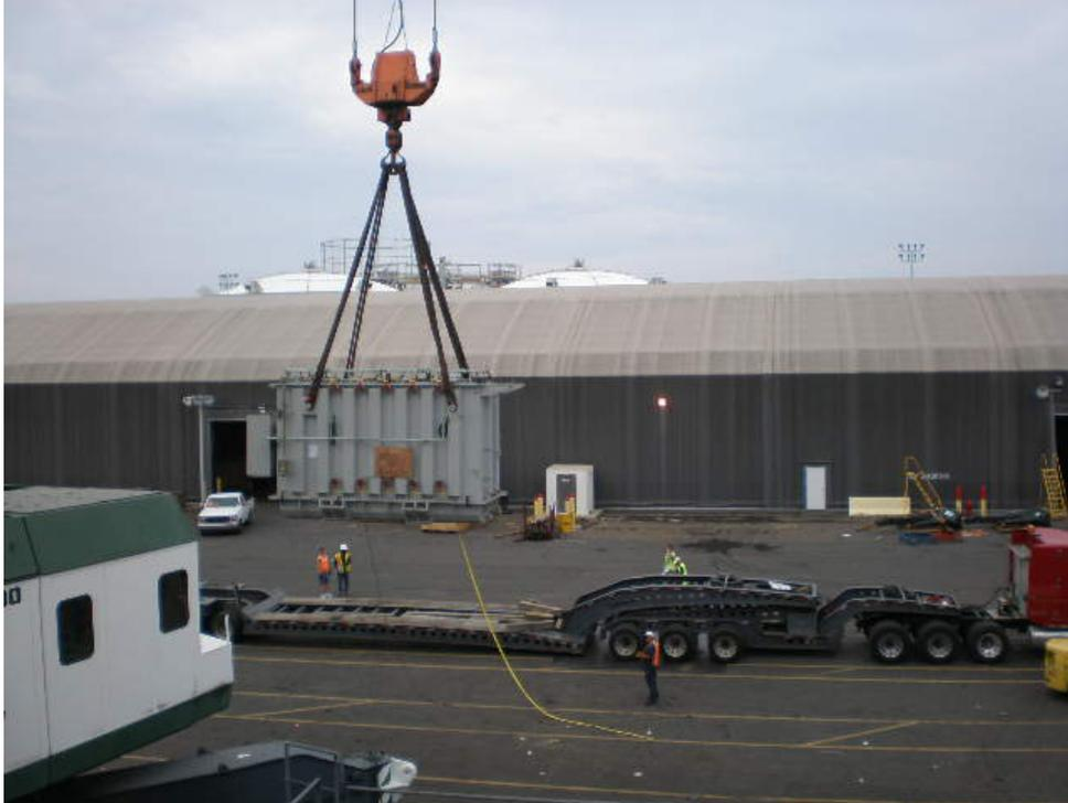
85 ton transformer is lifted from the ship's hold by the terminal shore crane and placed directly on a heavy haul trailer for transport to job site.
