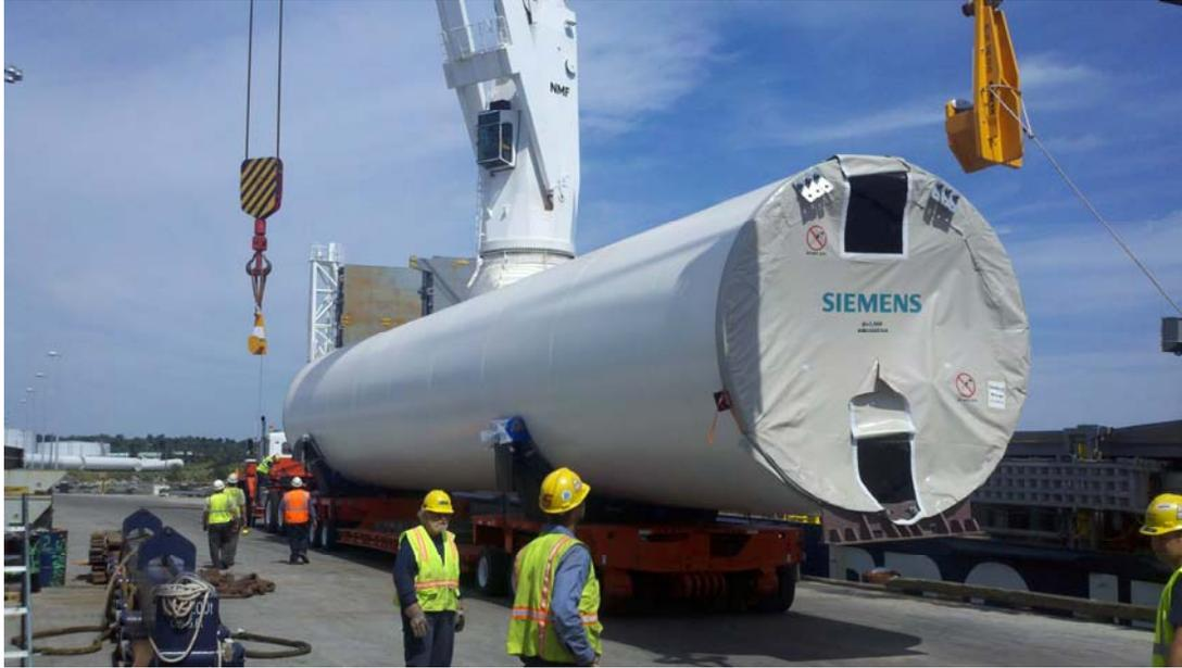
Tower section, shipped in a custom cradle, set atop trailer by two shore cranes, working in tandem. Below two power train & gear units are secured on mafi trailers for transport aboard a RoRo. Well marked lifting points are needed, as well as protection against the elements.
